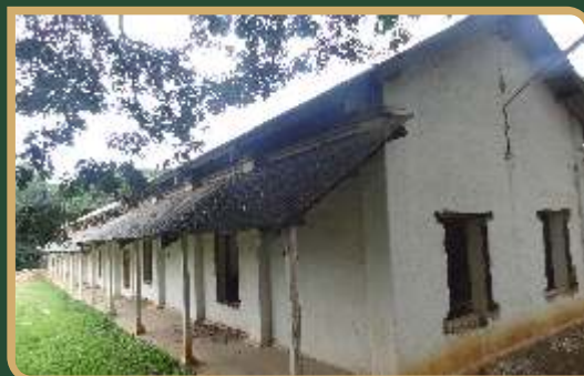
DEMOLITION DRIVE FOR DEPLETED OLD BUILDINGS
