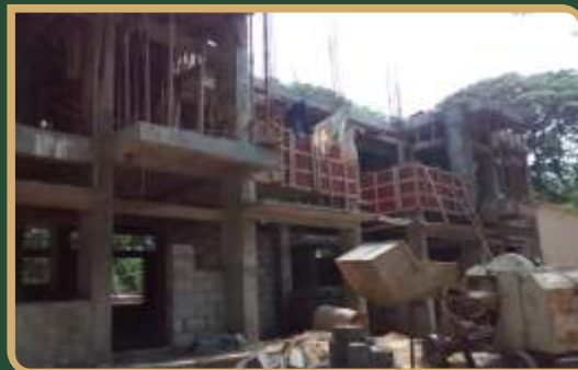
06 X QTRS FOR ASST MASTERS : UNDER CONSTRUCTION
