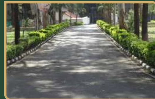
ROAD WIDENING ALONG WITH PAVEMENTS
