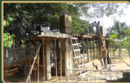
NEW REAR GATE WORK IN PROGRESS
